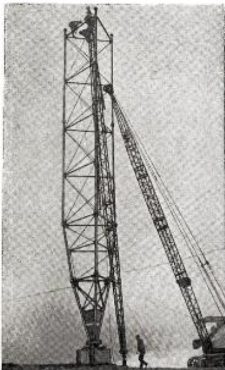
Construction close-up on new 1282-foot Truscon Triangular Guyed Tower for WWTV in Cadillac, Mich.
